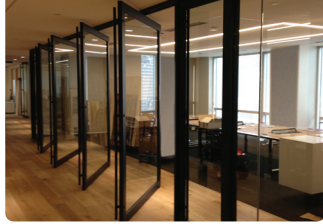
Total Vision Custom Pivot Interior Doors 1/4" x 6-ft. wide doors complete with pivot Glazing Contractor: Eastside Glass
